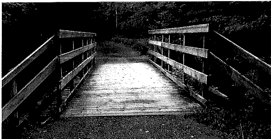
Figure 4-5: View of Rail Corridor Bridge at Black's Brook
