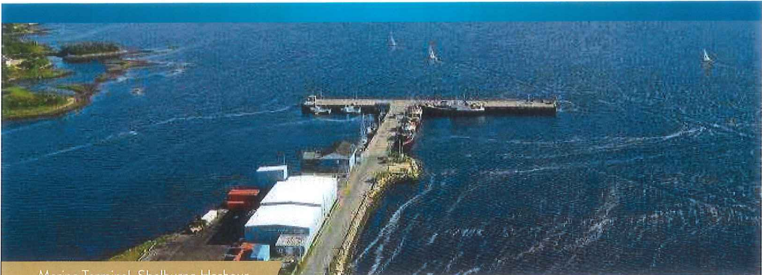
Marine Terminal, Shelburne Harbour
